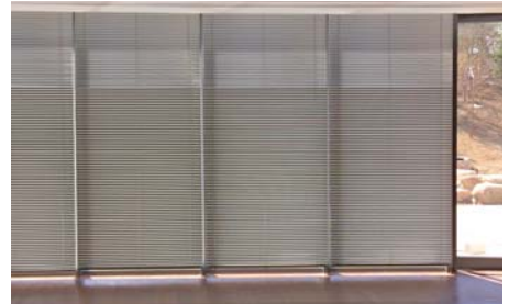
Fig. 12: Apec, Yan Xi Lake Beijing, China; Arch.: BIAD Beijing Institute of Architecture, Beijing, China. During 90% of the occupied hours, the blinds remain in a horizontal position.
