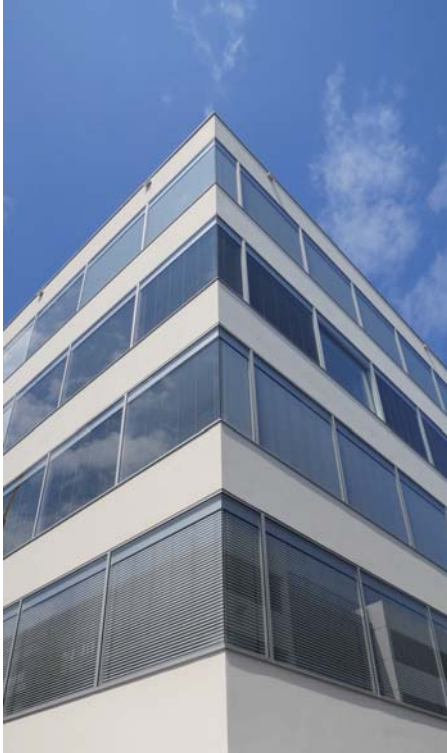
Fig. 31: New construction Analytical Laboratory, Kaiseraugst, Switzerland; Owner and Occupant: Hoffmann-LaRoche AG, Basel, Switzerland, Arch.: Nissen & Wetzlaff Architekten, Basel, Switzerland; Main Planning: Itten + Brechbühl AG, Basel, Switzerland; Facade construction: Gartner; Daylighting: Köster Lichtplanung, Frankfurt a.M., Germany
