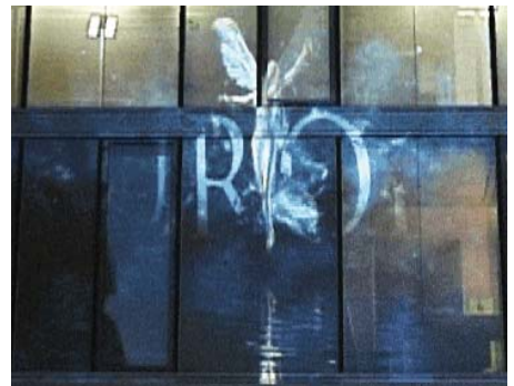
Fig. 25: Media façade with RETROLuxTherm projection onto the white lower surface of the louvers.
