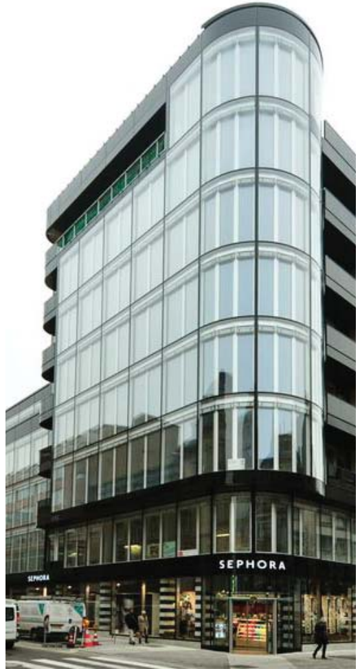
Fig. 30: RUGO, Luxembourg-Ville, Luxembourg. Non-ventilated double-skin, partly rounded façade with segmented RETROFlex blinds. Arch.: BALLINIPITT, Luxembourg.
