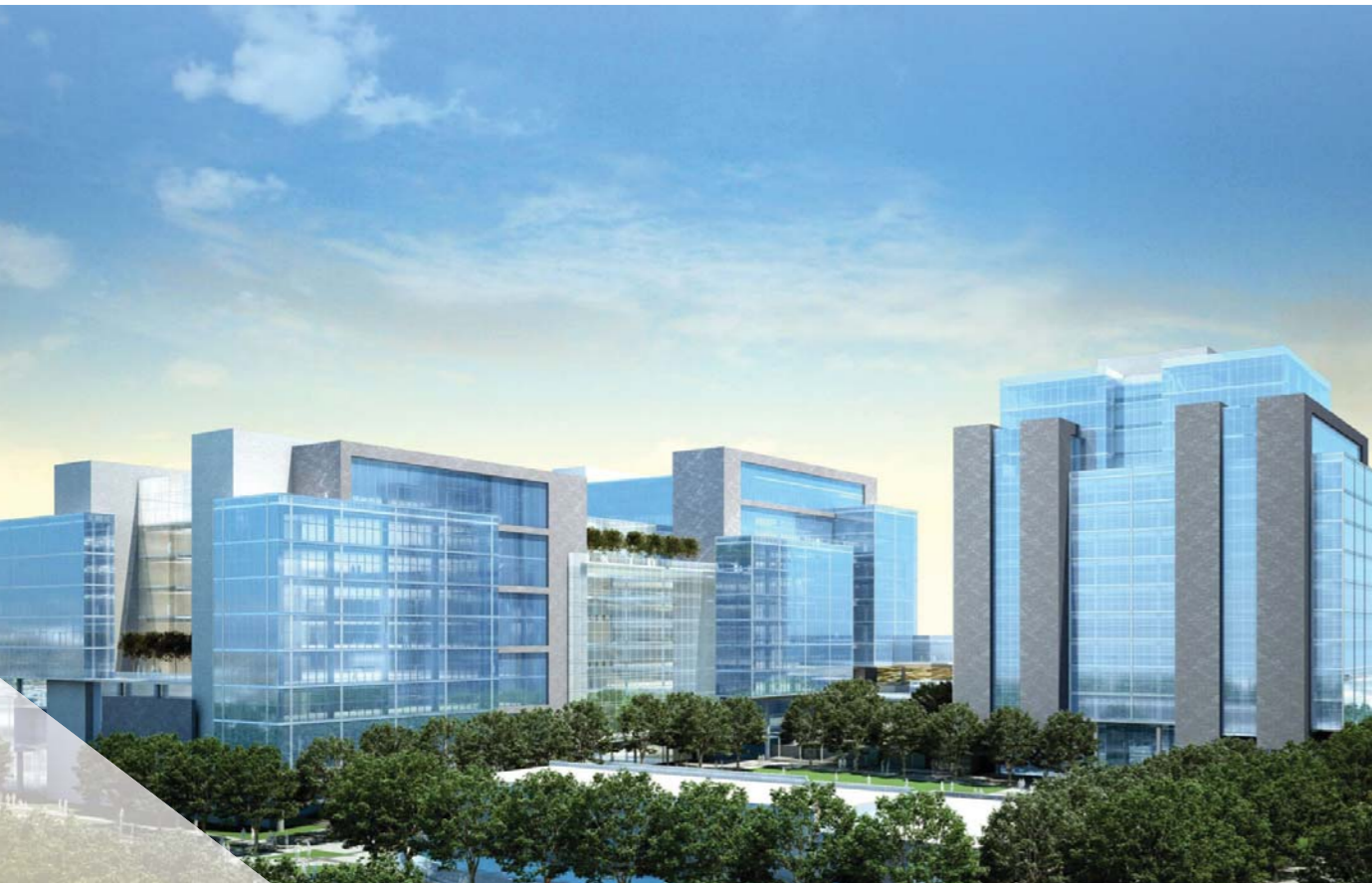
Standard Bank, Johannesburg, South Africa Architects: GLH, Associate Architects, Grosskopf Lombard Huyberechts, Johannesburg Façade construction: PURE, Neil MacLeod, Johannesburg Electro technique: Claassen Auret Inc., Johannesburg HVAC: Craig Cumming, Johannesburg
