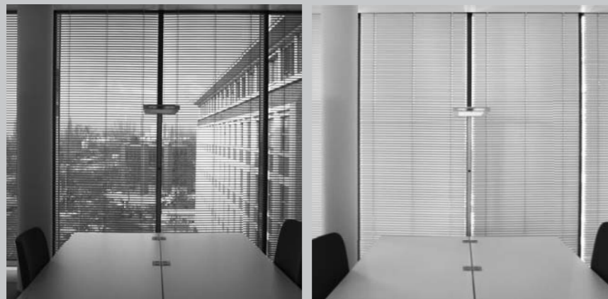
RETROLux in Sonnenschutz- und Abdunkelungsposition RETROLux in solar protection position and closed position
